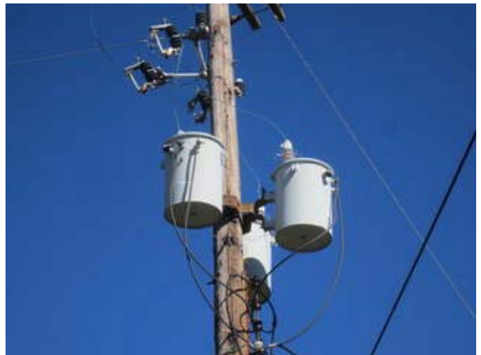
Pole Mounted Transformers
