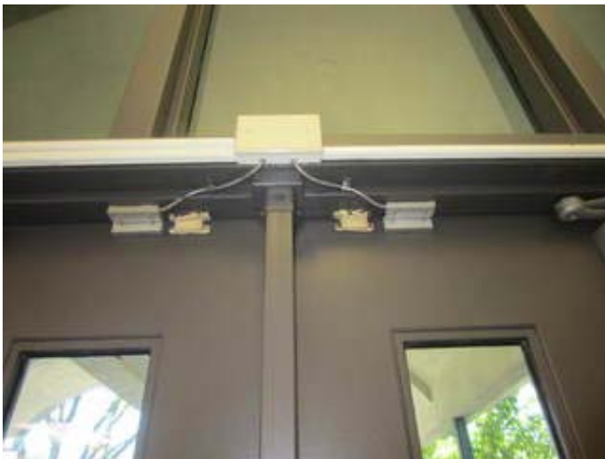
Security System Door Contacts
