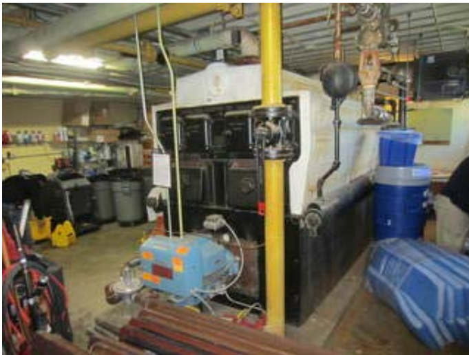
Natural Gas Fired Heated Water Boiler
