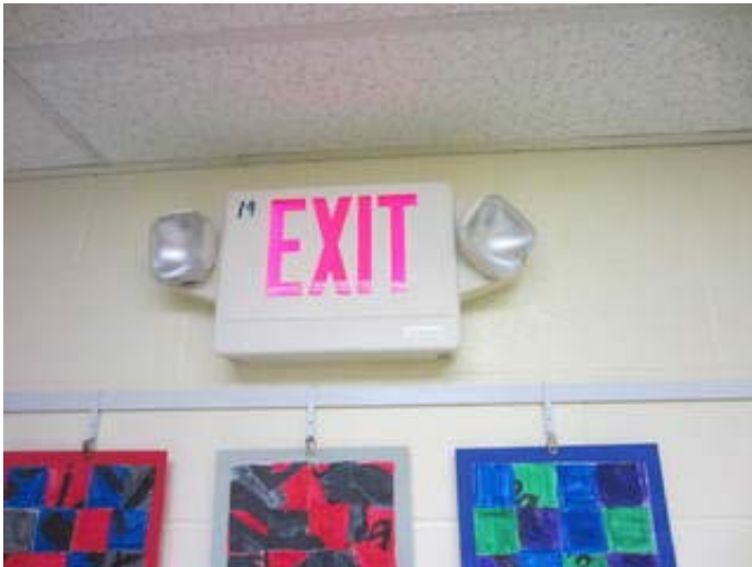
Exit Sign with Emergency Egress Lighting
