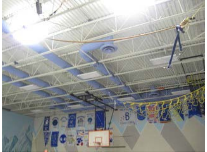
Steel Joist Structure
