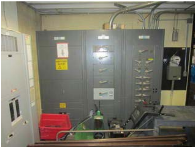
Main Electrical Distribution Panel
