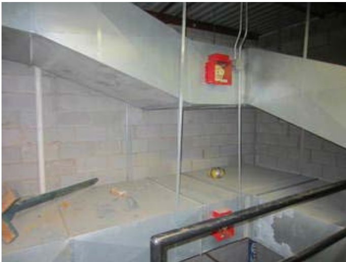
Fire Alarm System Duct Detector
