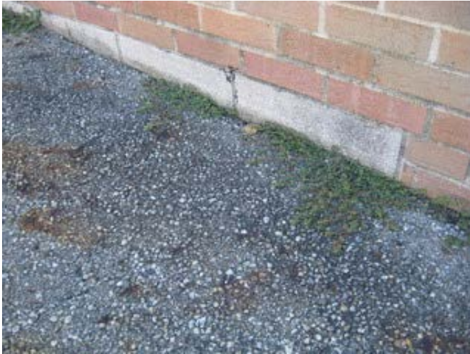
Concrete Masonry Foundation Wall
