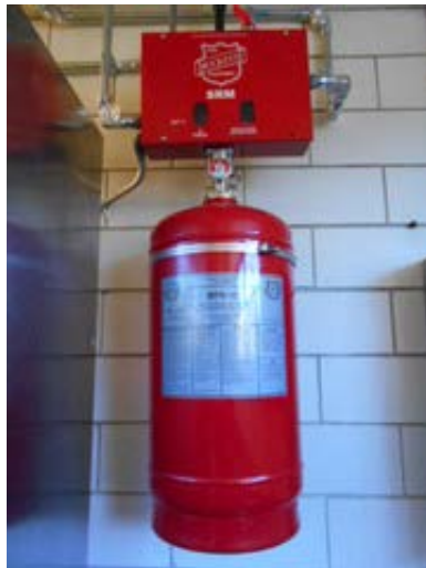
Compliant Wet Chemical Fire Suppression System-1964 Original Construction
