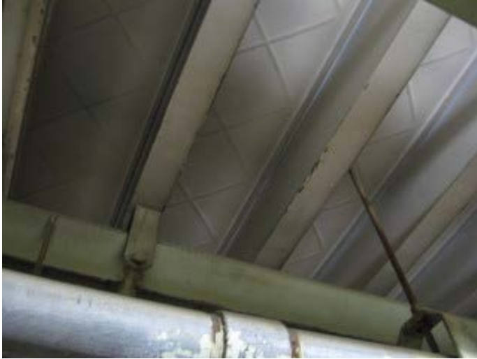
Preformed Composite Structural Metal Deck
