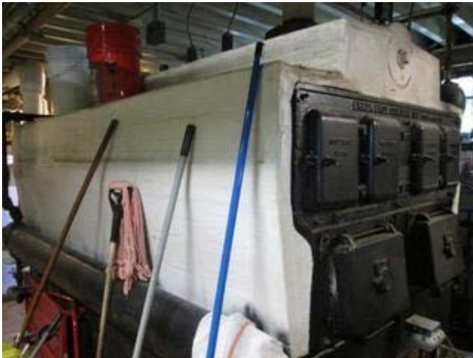
Boiler Insulation
