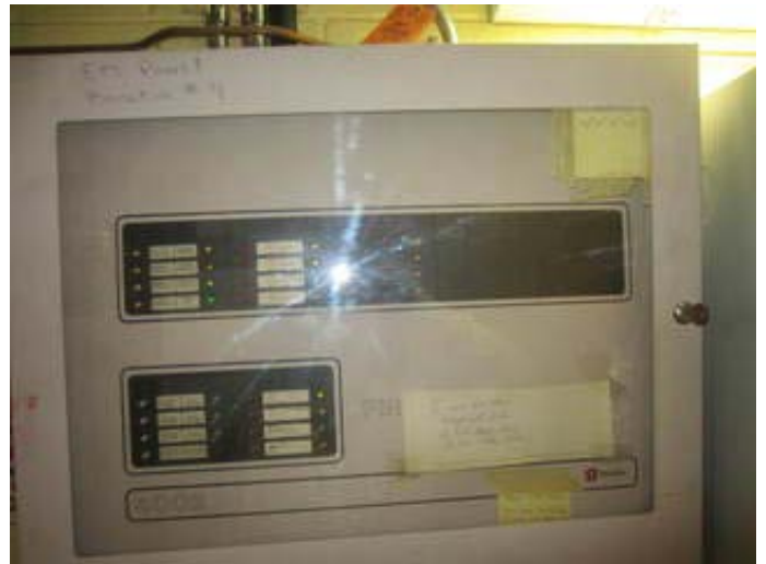
Fire Alarm System Control Panel
