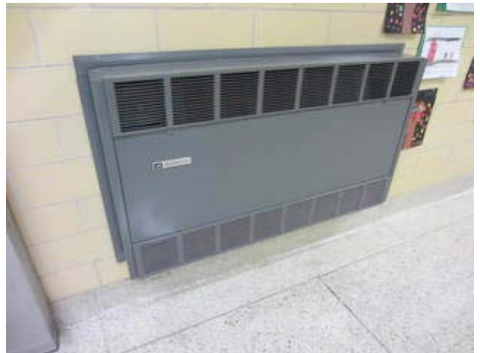
Heating Water Cabinet Heater
